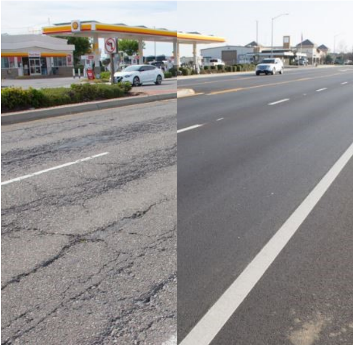
“Before” and “after” pictures from the resurfacing of State Route 113 in the Solano County community of Dixon.
